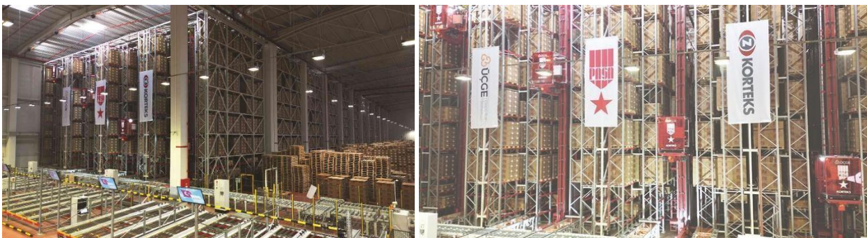
Figure 31. Korteks Automated Warehouse
